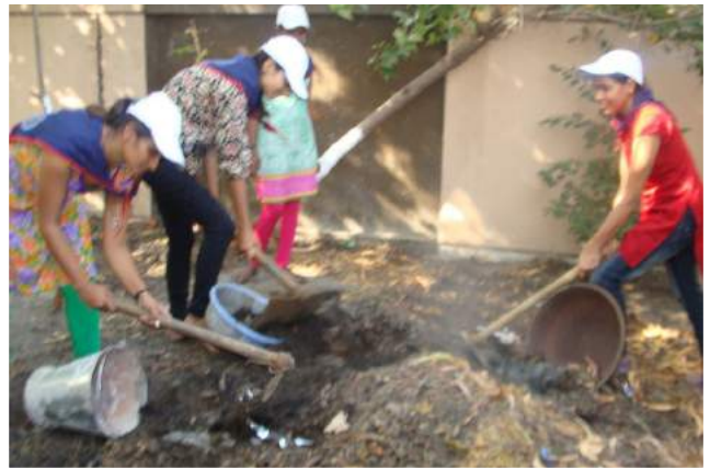
SHARAMDAAN - LEVELLING OF GROUND
